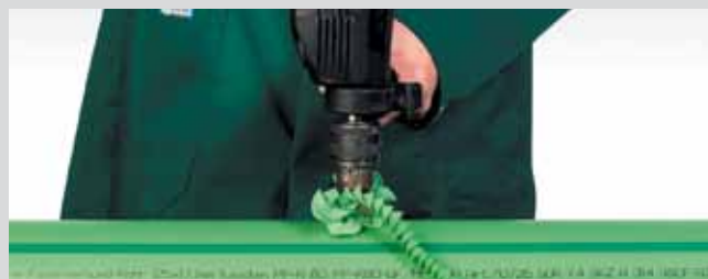
Drilling through the pipe wall
