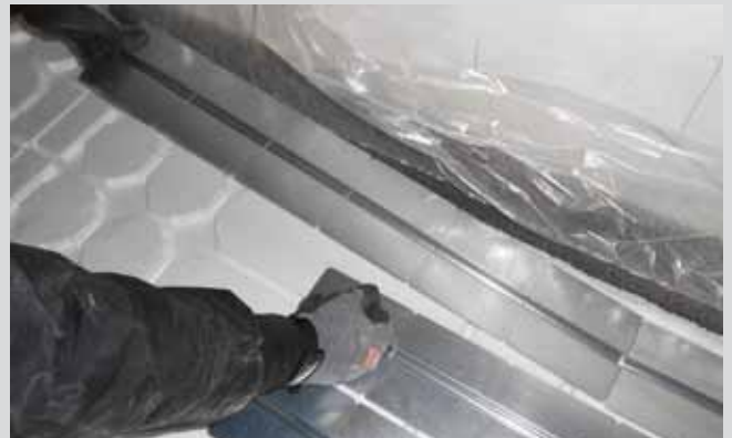
Installation of heat conducting steel sheets
