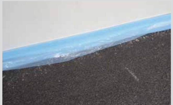
Laying of edge insulation
