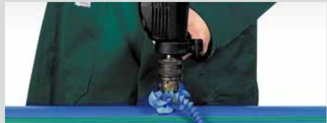
Drilling through the pipe wall
