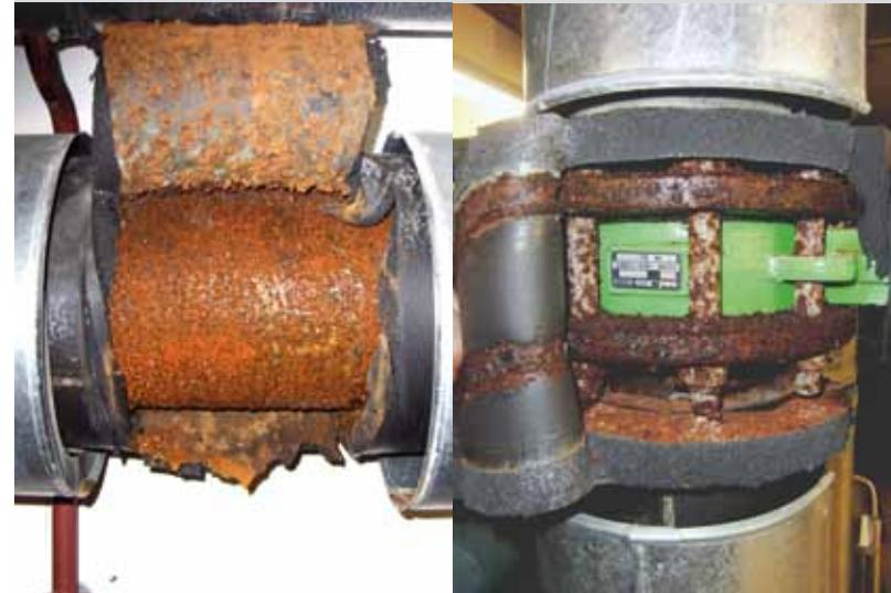
corroding steel pipes
